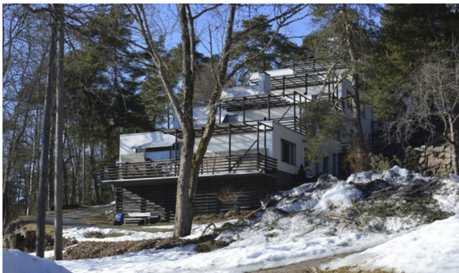
1. Terassitalo. Exterior view from southeast, looking up the steep slope. March 21, 2022, 13:41 © author.
