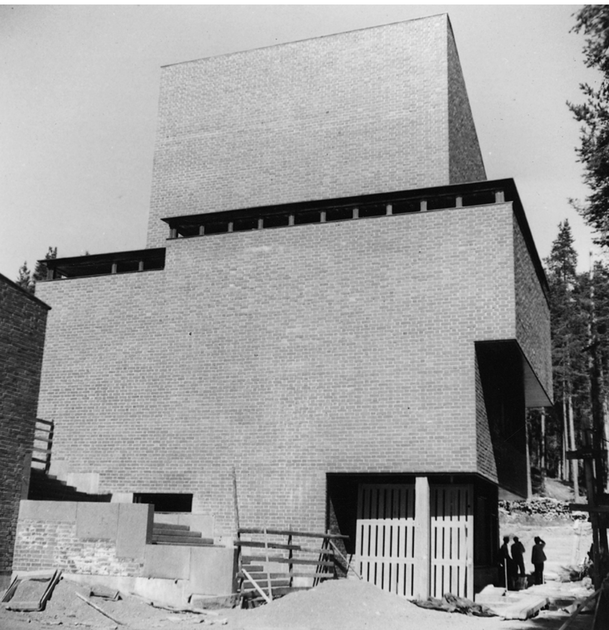
2. The town Hall under construction.
