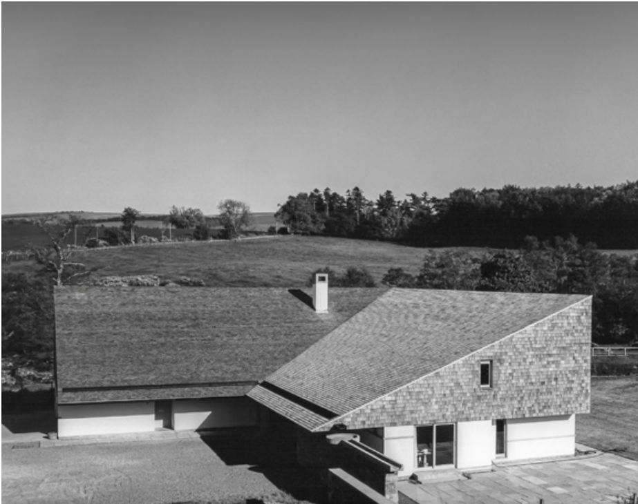
5. Exterior of the Balfour House Photo: © Morris and Steedman Associates
