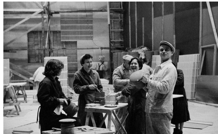
The construction of the House of Culture, men and women doing voluntary work in 1958. Photo: Väinö Kannisto, Helsinki City Museum
