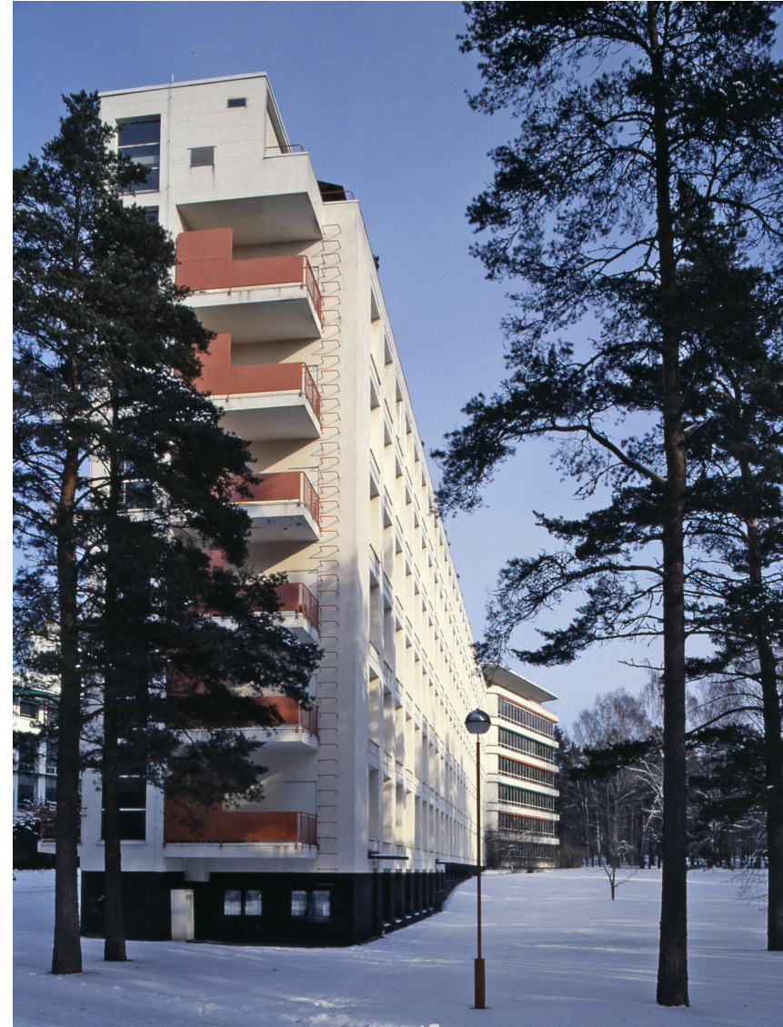
Paimio sanatorium main building, patients wing end with balconies and integrated fire escape stairs in 2007. Photo: Soile Tirilä, Finnish Heritage Agency
