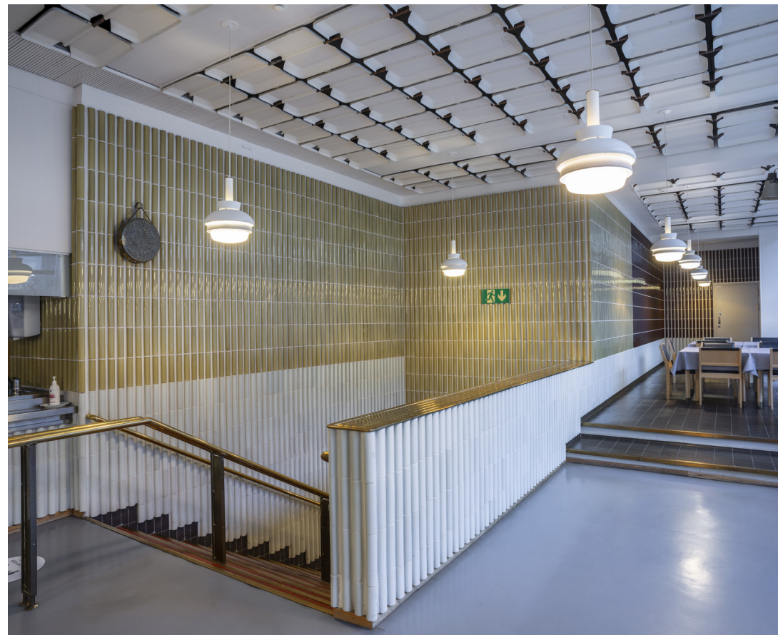
Ceramic clincker rods and light fixtures in the canteen staircase are designed for the Social Insurance Institution Main Office. The canteen in 2022. Photo: Maija Holma, Alvar Aalto Foundation
