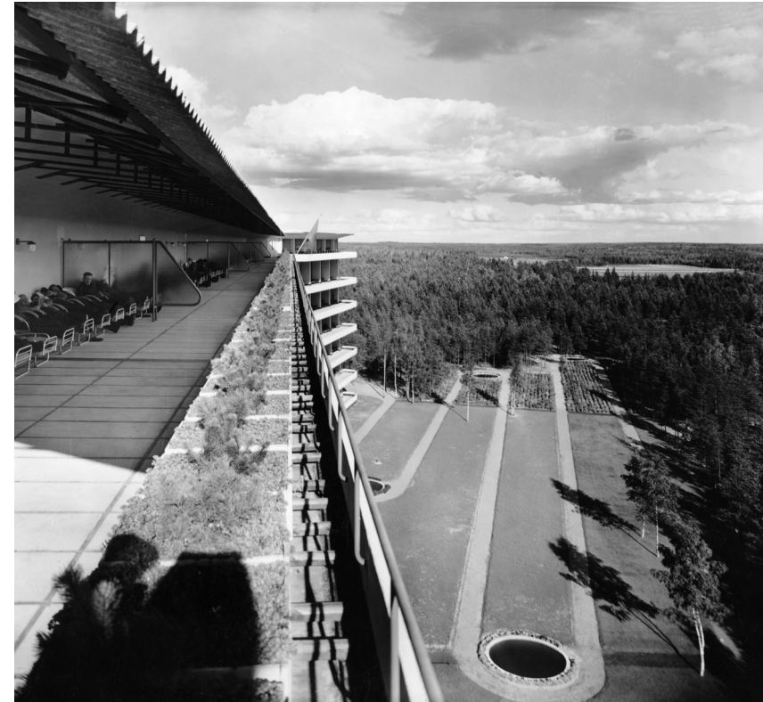
Paimio sanatorium solarium terrace in 1934. The roof strip was added to protect the patients from rain. Photo: Gustav Welin, Alvar Aalto Foundation.
