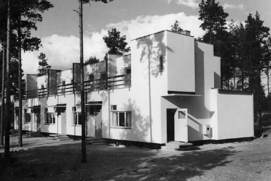
The completed staff housing (AAM 50-003-432 Gustaf Welin).
