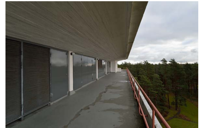
Roof terrace, 2015 (AAM Sakari Mentu)
