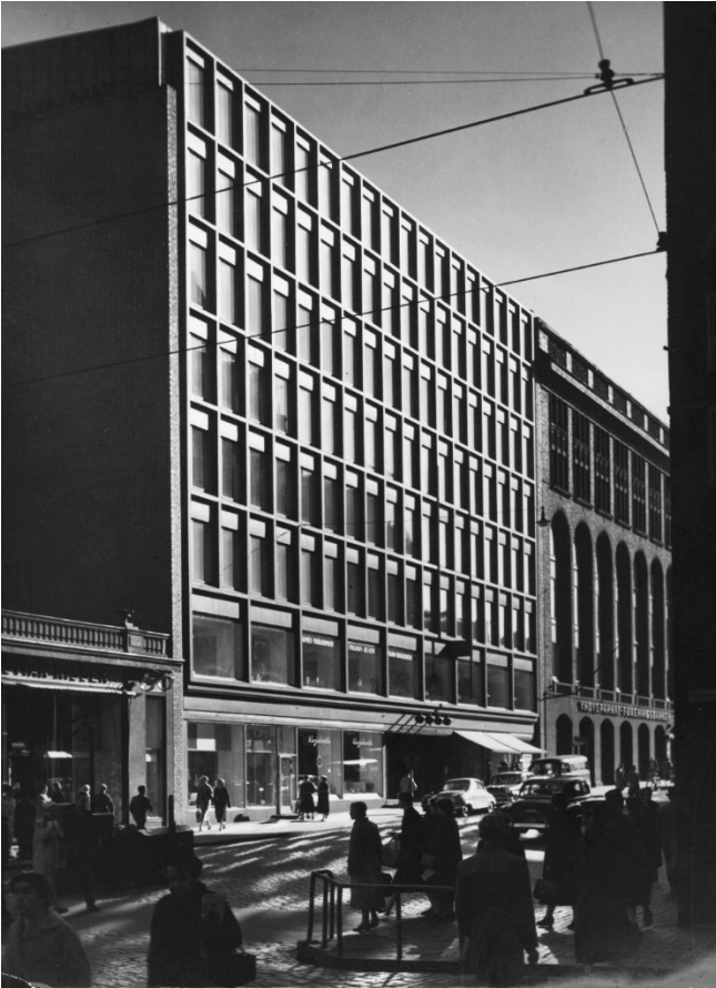
Fig 1. Rautatalo office building has a grid façade made mainly of copper sheets. Photo AAM.
