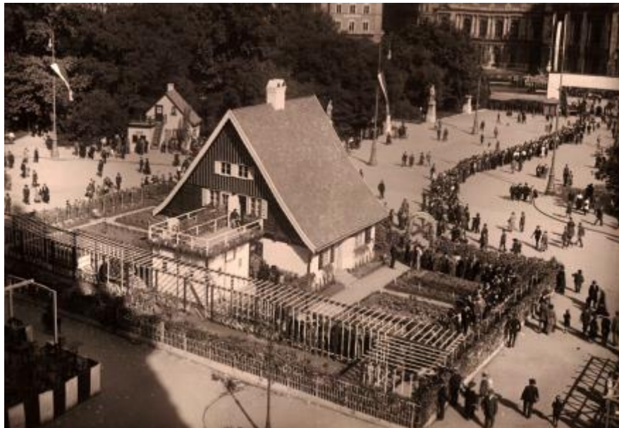
Figure 6: Visitors in front of Vienna's 1923 Allotment Garden Settlement and Housing Exposition, lining up to see Burgenland Type.
