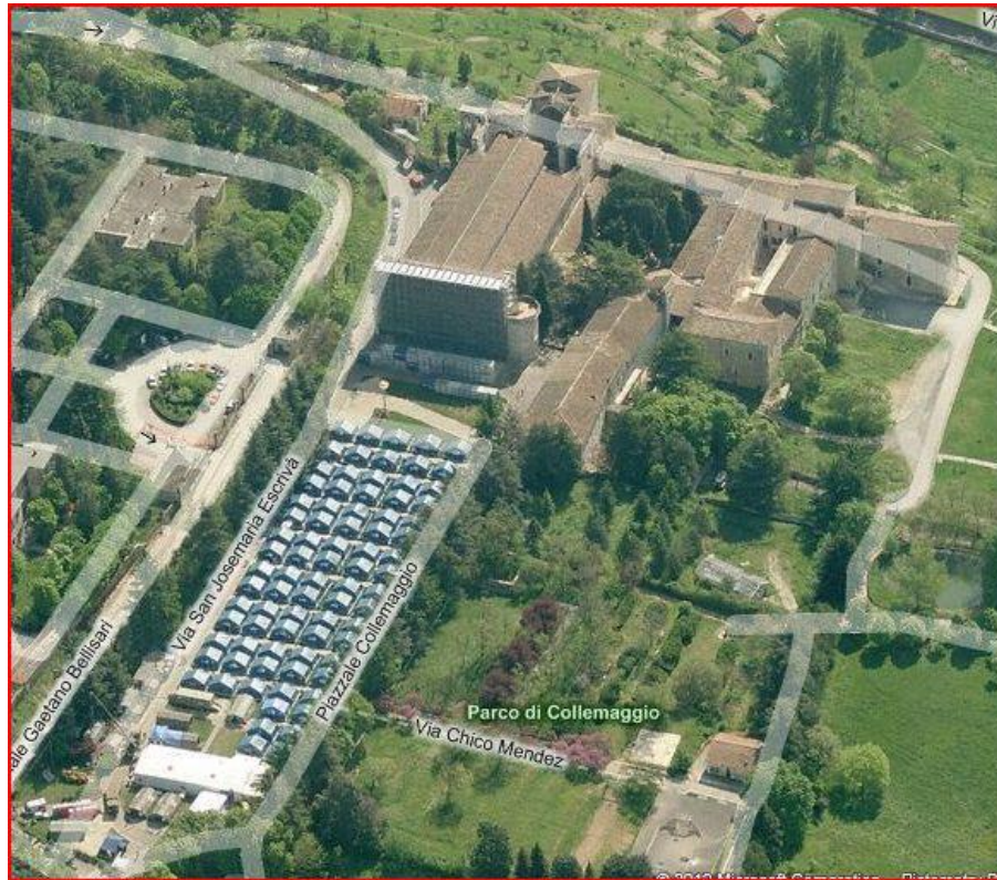
Fig. 5: Aerial photo of the first tents camp located in front of Santa Maria di Collemaggio cathedral after the 2009 L'Aquila earthquake.
