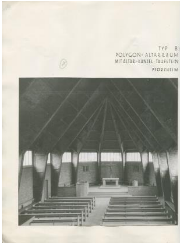
Figure 7: Otto Bartning, wood structure prefabricated church, 1946-50. Source: ©Otto Bartning Archiv, TU Darmstadt
