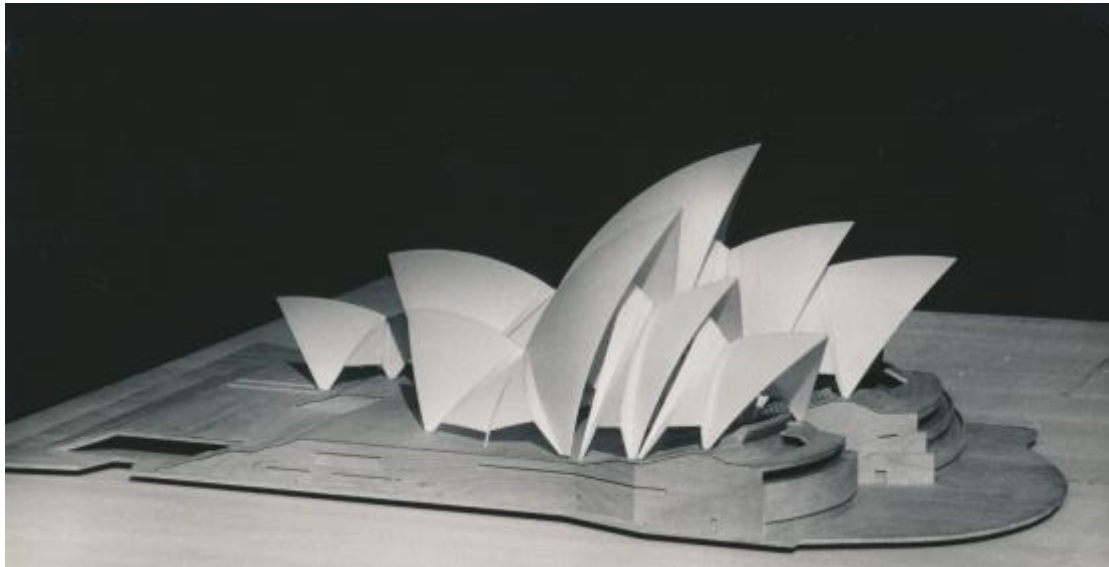
Figure 6 Utzon's 1962 model showing the iconic roof/earthwork juxtaposition of the Sydney Opera House and its finalized shell-vault structure of roof forms. The Utzon Archives , Aalborg University Library.
