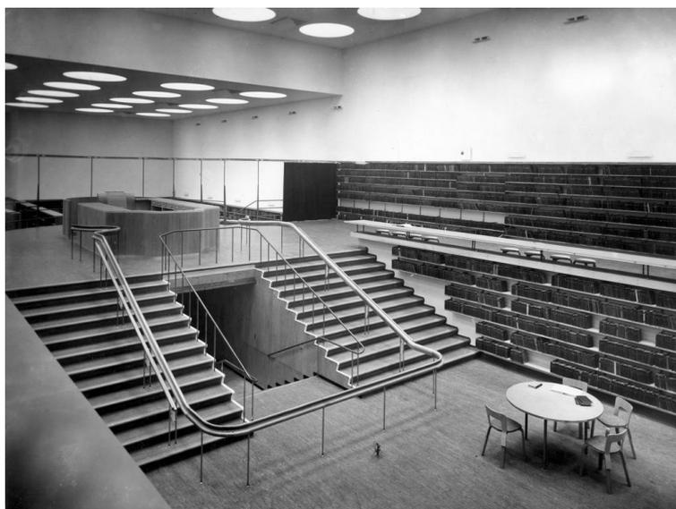
*Viipuri City Library (Viipuri, Finland 1935). Reading rooms and book collections are connected with staircase. Handrail separates a route for visitors. An ideal diffuse illumination for reading is obtained by placing light sources – the 'many suns' – deep into the circular cylinders. Photo: Alvar Aalto Museum*
