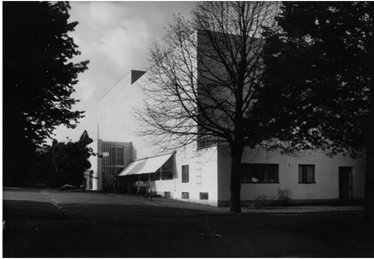
Vyborg Library 1935. Sun shades over the windows. In addition to mechanical and electrical systems in his architecture, Aalto used also traditional passive methods to control the indoor climate. Photo: Alvar Aalto Museum.
