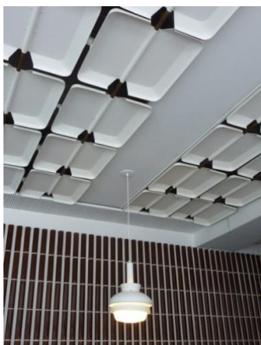
Concave shaped, white aluminium plates were manufactured by Oy Sohlberg Ab in Finland. Photo Seija Linnanmäki 2012.
