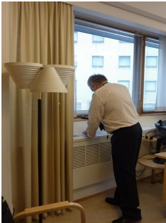
Office room with Carrier Weathermaster fan coil unit under the window sill. Original system is restored and still in use. Photo Seija Linnanmäki 2012.
