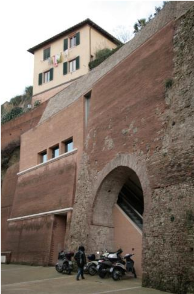
ill. 2 – The exterior of the escalator at Fontebranda in the city centre of Siena. The exterior walls were built so that the new structure would merge with the stones and bricks of the surrounding buildings and walls. Photo credit: by the author.
