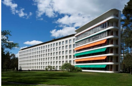
Paimio Sanatorium, patients' wing and solarium terraces. Photo: Maija Holma, Alvar Aalto Museum
